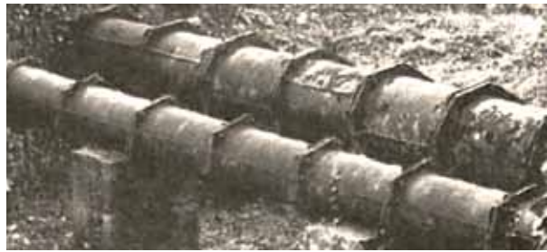
This gray cast iron pipeline was in service for more than 330 years. Today such pipes are manufactured from ductile iron. Ductile iron possesses all excellent properties of gray cast iron. Furthermore it has much better mechanical properties.
