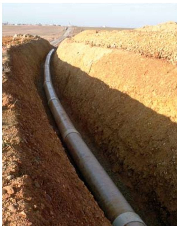
Figure 12-7 Flowtite coupling, angular joint deflection
